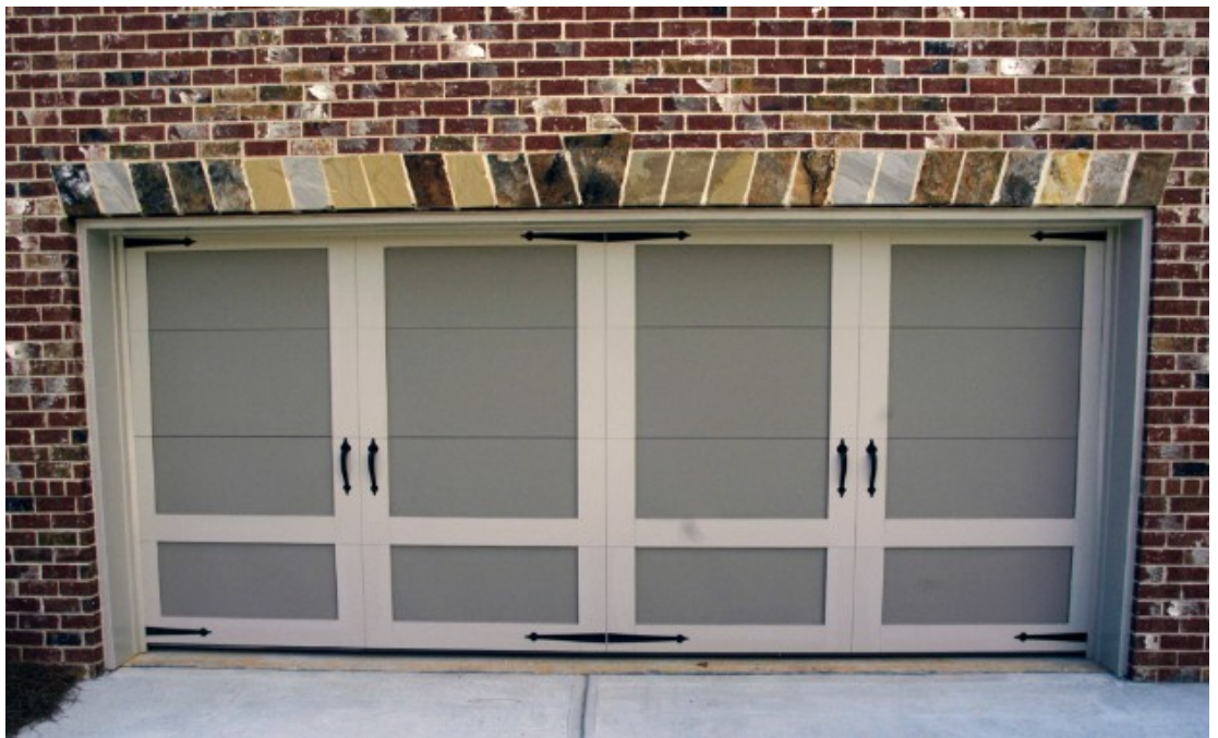
2 sets of hardware on this door
